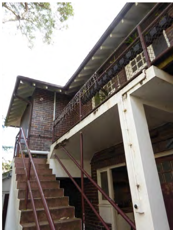
Rear stairs and landings of concrete with pipe rails
