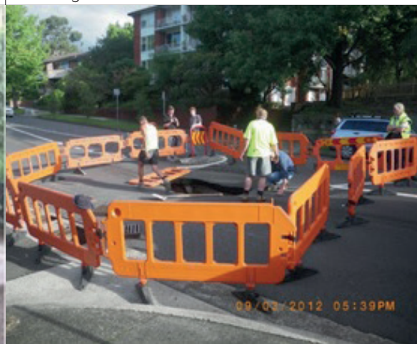
Sink hole in road near pipe
