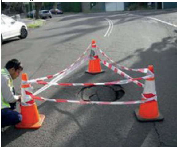
Sink hole in road near pipe
