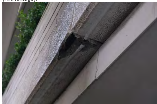
Figure 14: Example of damaged concrete caused by corrosion of steel reinforcement (RKHeritage).
