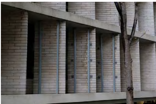
Figure 13: Example of steel bracing fixed to damaged sunshade fins (RKHeritage).
