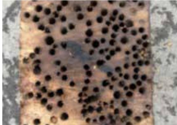
Evidence of marine worms in timber structure
