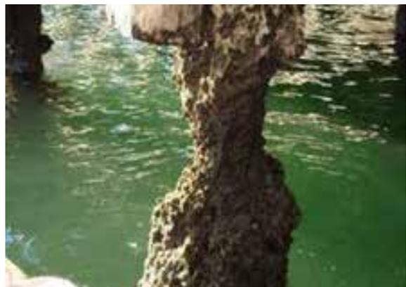
Beams and girders in very poor condition
