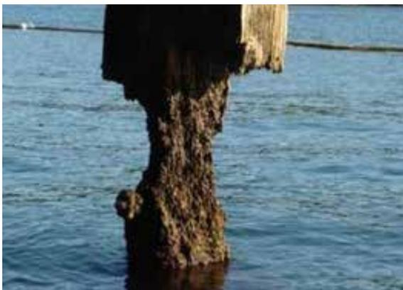
Pile in very poor condition
