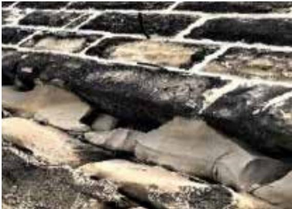
Blocks missing and eroded
